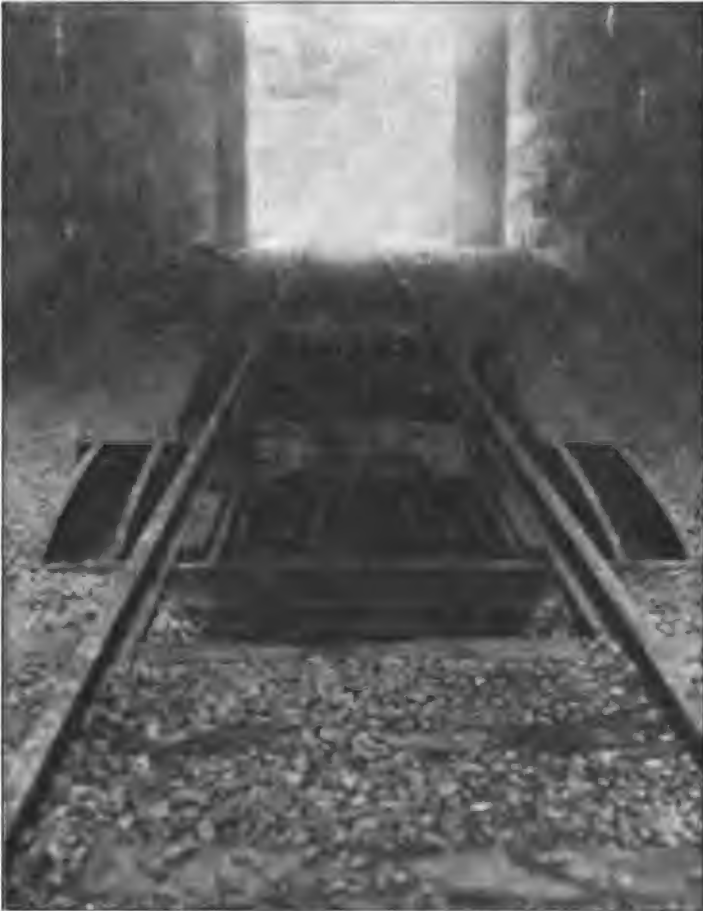
INTERIOR OF CONCRETE EMPLACEMENT FOR 340-MM. FRENCH GUN (LOOKING TOWARD THE ENTRANCE).
